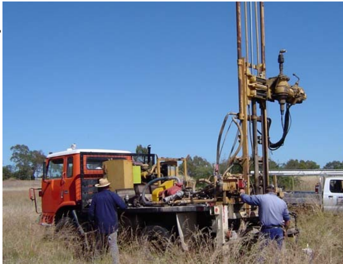
Drilling the extraction bores on the site
